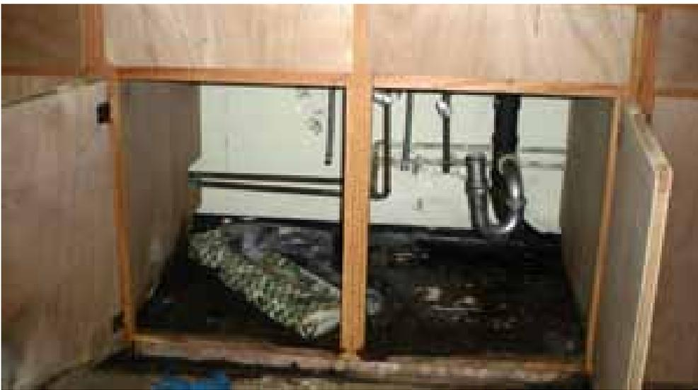
Damaged wooden cabinets due to mold.
