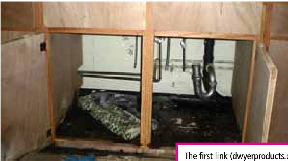
Damaged wooden cabinets due to mold.
